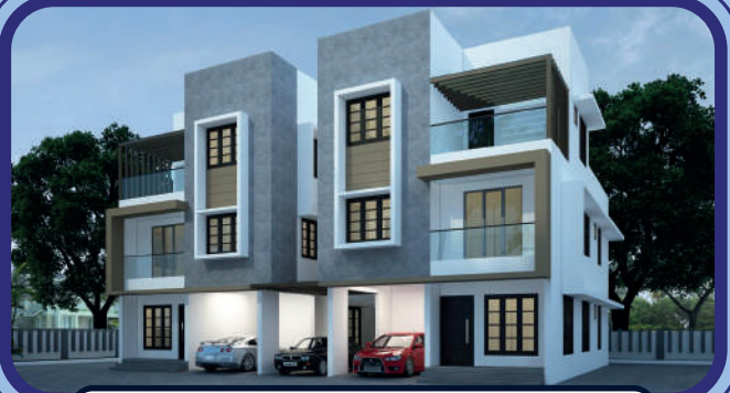
Residential Building consisting of 3500 Sqft. costing Rs.1.5 Crore at Carmelaram.(Joseph) 2020
